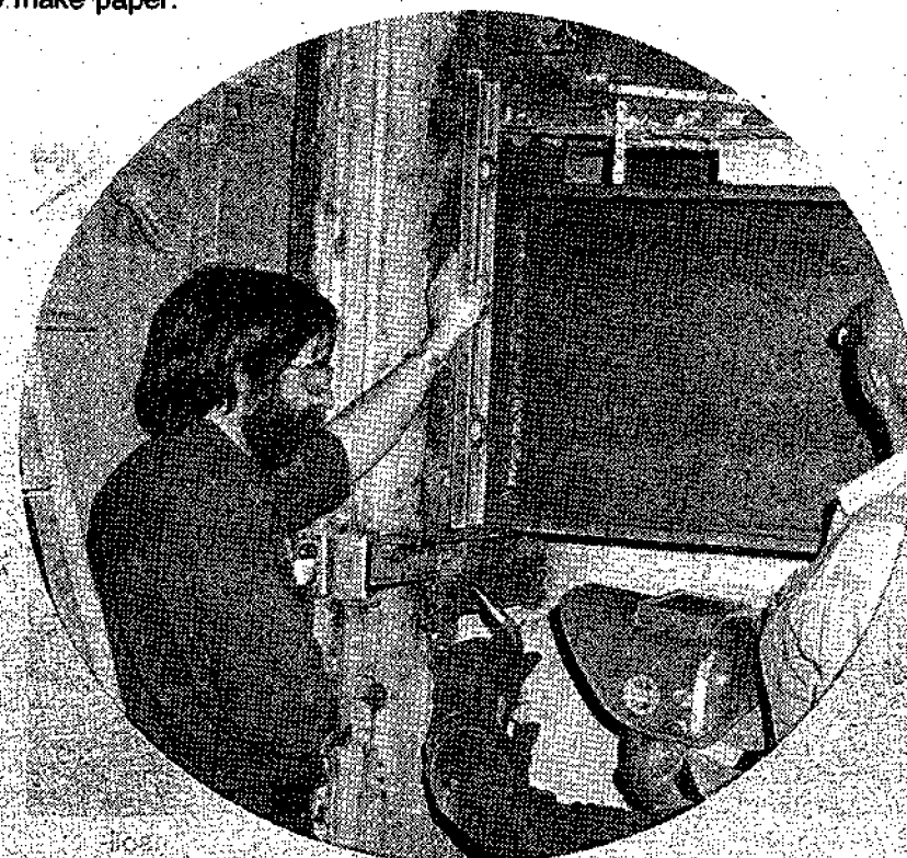
Teamwork —Millwrights Rodney Breit and Charlie Huisheere check for proper placement of a large beam while welder Denis Kester prepares to tack it in place.
